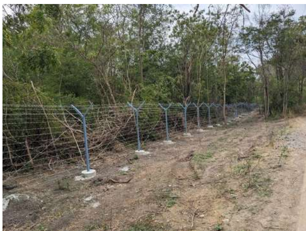
The IIT fence work going on at Annapurna Farm....
