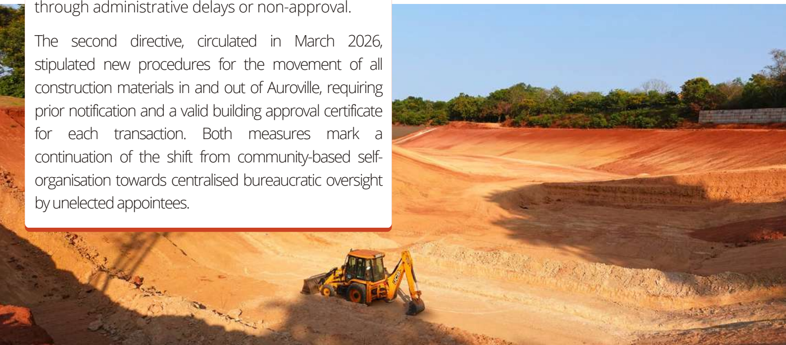
Digging the Matrimandir lake, April 2026
