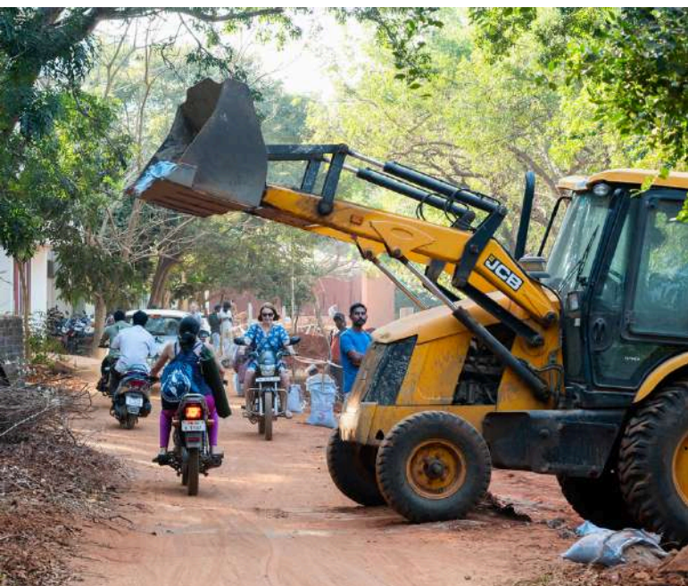
Ongoing works on the Vikas radial, February 2025
