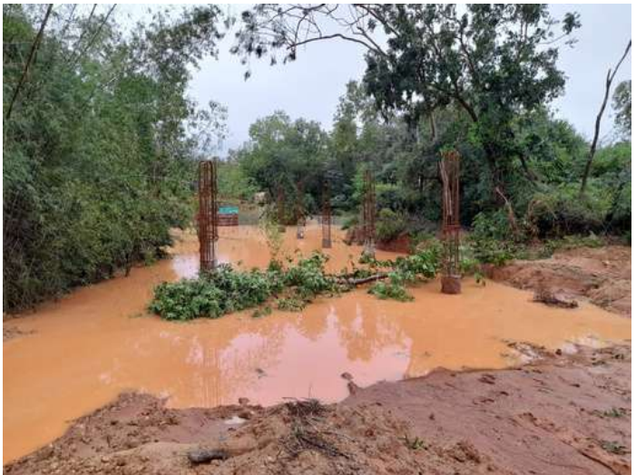
Bridge under construction through Darkali watershed
