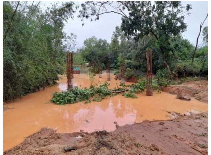
Bridge under construction through Darkali watershed
