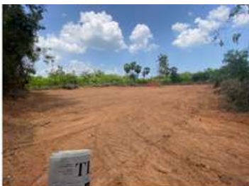
Figure 3 Overview of site
