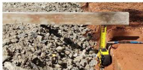
Fig. 70: Course higher by 8 cm above old road level
