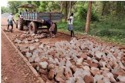
Fig. 58: Transportation of pavers
