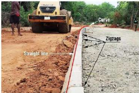
Fig. 26: Zigzags and kerbs linear and not curved
