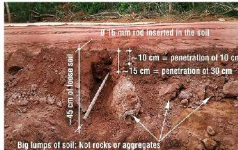
Fig. 17: Bottom part of the layer not compressed
