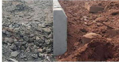
Fig. 21: No plain concrete on the sides
