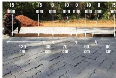
Fig. 26: Waves in lengthwise before ramming
