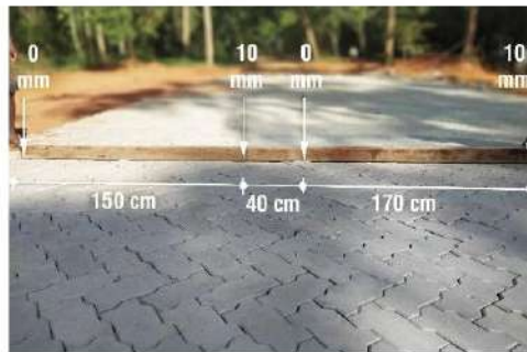
Fig. 21: Crosswise levelling before ramming
