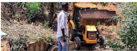
Fig. 5: Taking away small wood, branches and roots
