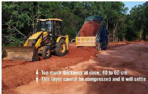
Fig. 14: 40 to 60 cm of loose red soil at once = far too thick
