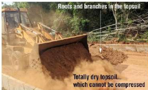
Fig. 3: Pushing dry topsoil
