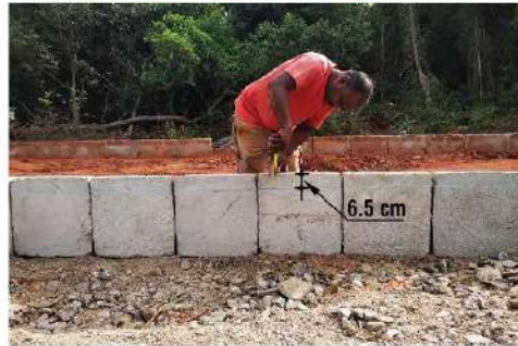
Fig. 33: Inaccuracy of levelling
