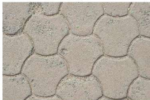
Fig. 61: Texture of pavers after 12 years & 14,864 mm rainfall
