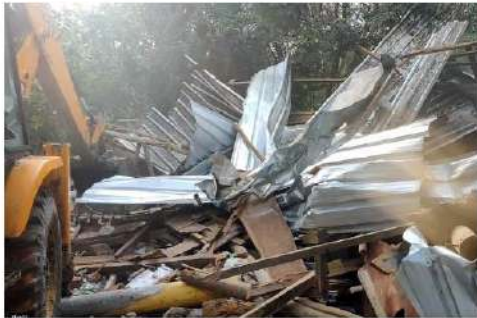
Fig. 87: Demolition of game room without warning and with all things inside
