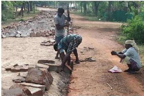
Fig. 56: Removing the kerbs
