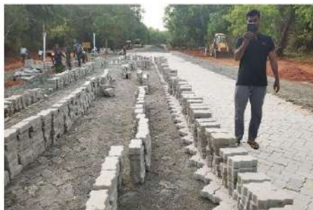
Fig. 3: About a quarter of pavers removed
