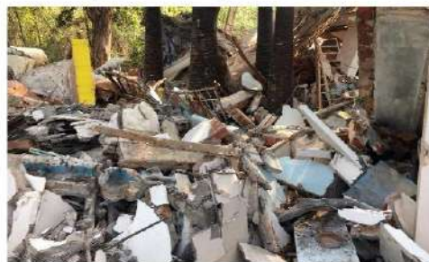
Fig. 97: House of Tapas destroyed
