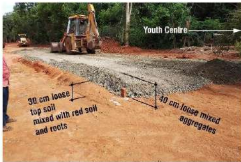
Fig. 11: In front of YC: filling with red soil mixed top soil
