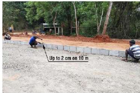
Fig. 27: Kerbs not levelled, up to 2 cm difference
