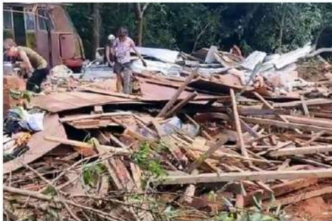
Fig. 89: Kitchen destroyed without notice and with all things inside
