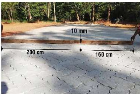
Fig. 22: Crosswise levelling before ramming
