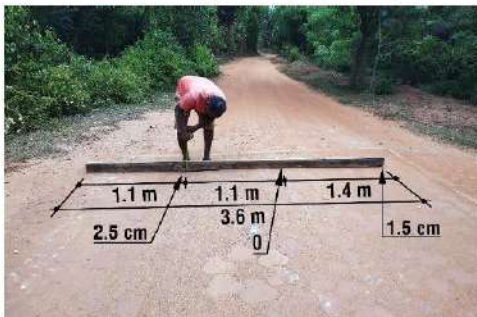
Fig. 64: Existing road at Kalabhumi
