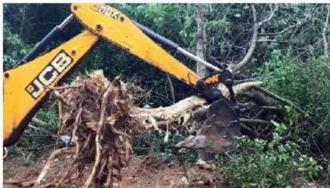
Fig. 92: Bulldozing old trees at Darkali
