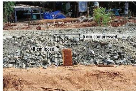
Fig. 12: Single layer of mixed material of 40 cm and not 10
