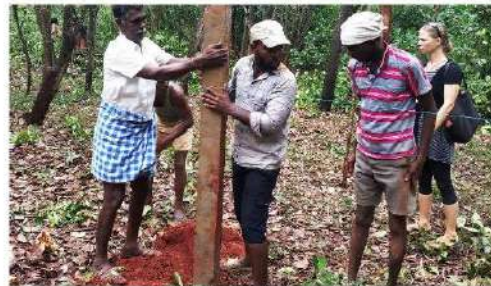
Fig. 2: Workers laying posts
