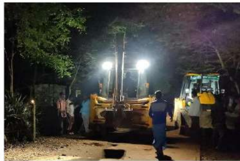
Fig. 80: JCB bulldozing at night with police force
