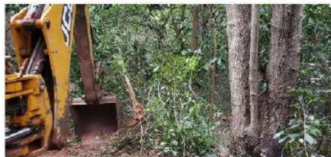
Fig. 2: Bulldozer opening a cycle path
