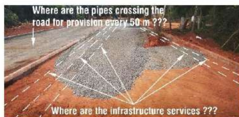
Fig. 5: No service laid... but pavement is being prepared
