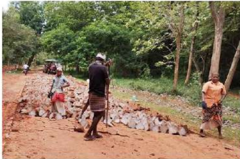
Fig. 54: Removing pavers which are in a very good condition
