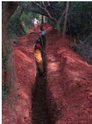
Figure 5 – Trench for HT line in Auroville International Zone – Overview
