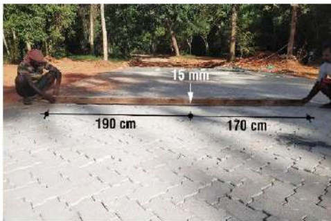
Fig. 20: Quality of levelling (crosswise) before ramming
