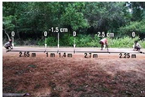
Fig. 65: Existing road at Gaia
