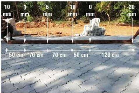
Fig. 24: Lengthwise levelling before ramming
