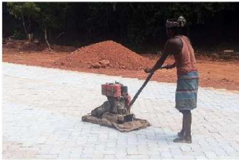
Fig. 10: Plate rammer to "level" the surface
