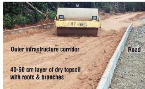
Fig. 4: Impossible to compress dry topsoil
