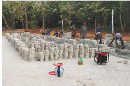
Fig. 2: Pavers removed during the night of the 13 th -14 th August
