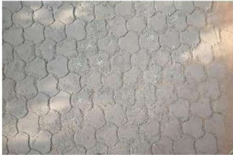
Fig. 62: Most damaged pavers at the entrance of Surrender Fig. 63: Most damaged pavers opp. Arka-entrance of Surrender
