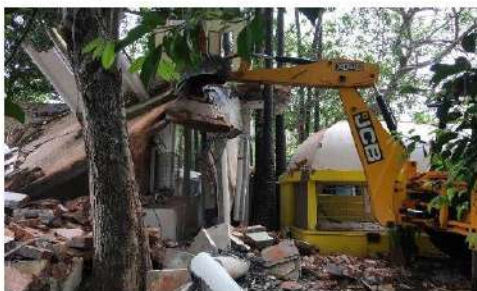
Fig. 96: House of Tapas being destroyed
