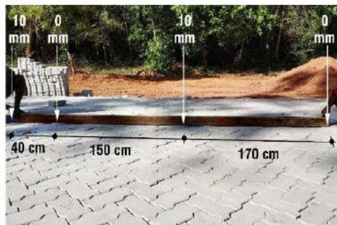
Fig. 23: Depressions in the length of the road, before ramming
