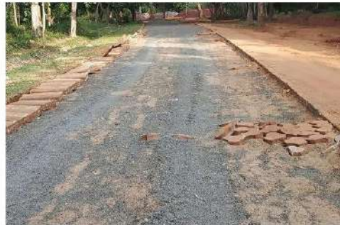
Fig. 59: River sand has been removed
