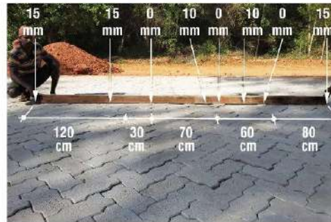
Fig. 26: Waves in lengthwise before ramming
