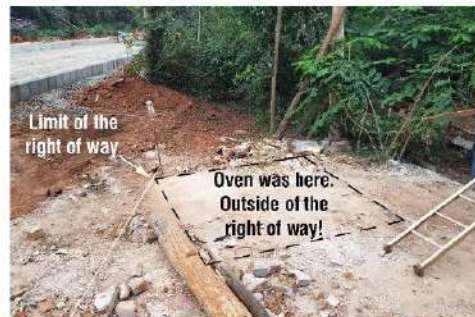
Fig. 9. Oven was outside of the right of way
