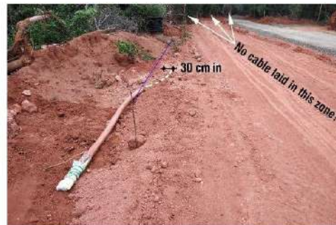
Fig. 41: Cable comes out in front, but no cable at the end
