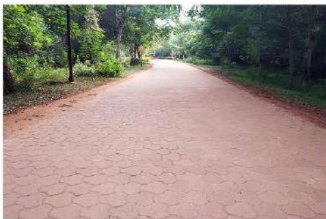
Fig. 60: Road after Arka, towards Gaia
