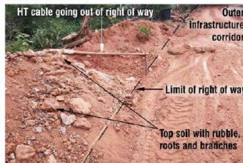
Fig. 9: Topsoil with rubble, roots and branches filling
