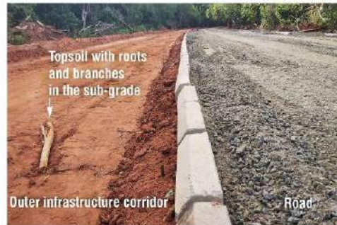
Fig. 7: Random alignment of the kerbs
