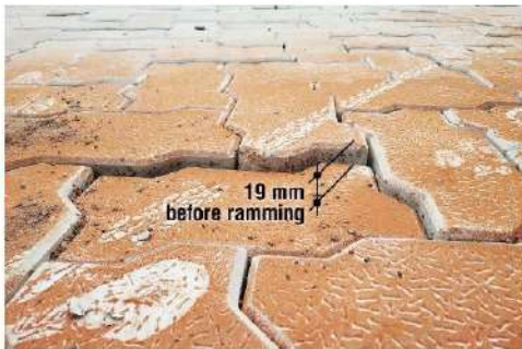
Fig. 16: Laying pavers = up to 19 mm before ramming
