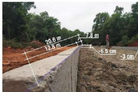
Fig. 31: Kerbs are not levels and show big bump
