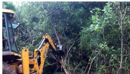
Fig. 15: Bulldozing trees at Darkali
